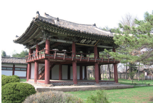
Figure Hamhung-I. Hamhung Royal Villa (Pavillion) (2012)
